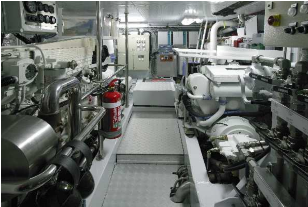
The engine room is laid out for excellent access to all machinery in a clean, bright and safe environment.
